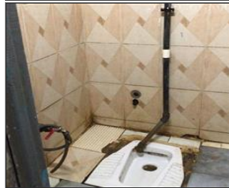
Photo of the sanitary facilities TOILET.jpg
