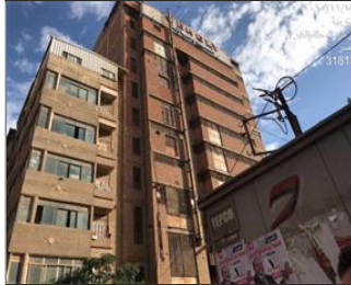
External photo(s) of the production unit(s) EXTERNAL PHOTO.jpg
